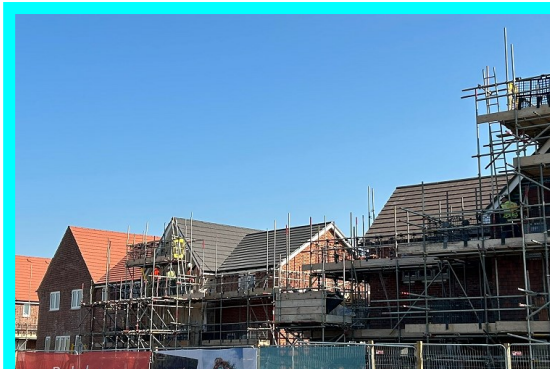
First homes under construction
