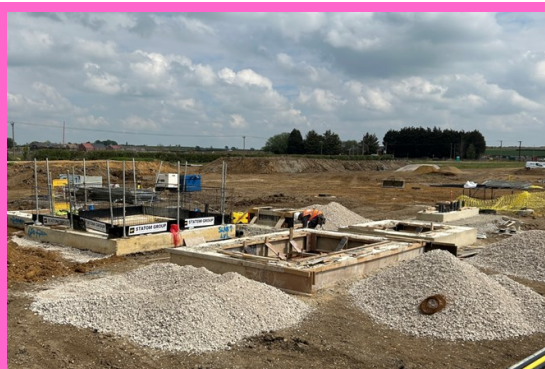
Pump Station 2—progressing well
