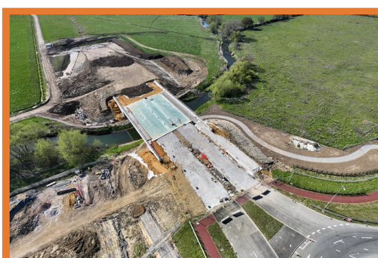
River Ouzel Bridge—good progress made
