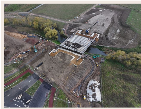
River Ouzel Bridge progress
