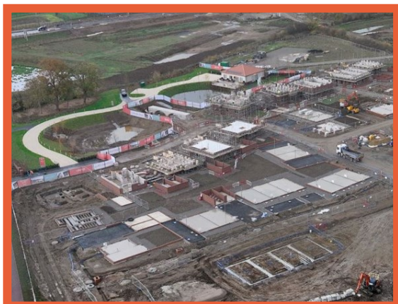
Phase 1A construction
